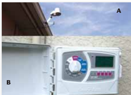
Fig. 1: The components of a Rain Bird ESP-SMT include A) the irrigation controller that replaces the timer and B) an independent weather station that replaces the rain sensor (still pictured) on the roof eave.
