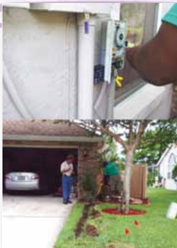
Fig. 2: The Baseline Watertec S100 soil moisture sensor was buried in the ground and the sensor controller was added to the current timer to bypass irrigation events when the soil was too wet.
