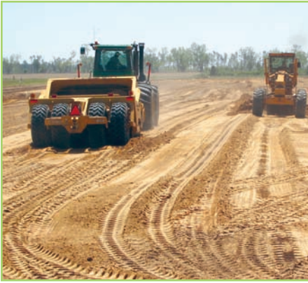
Fig. 1. Prior to the installation of the irrigation system, the topsoil was removed to a depth of 12" and stockpiled.
